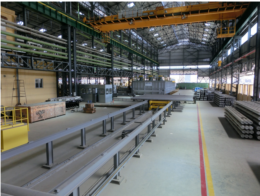
Continuous Homogenizing Furnace with log entry store magazine (foreground) and the homogenising furnace (Background)
