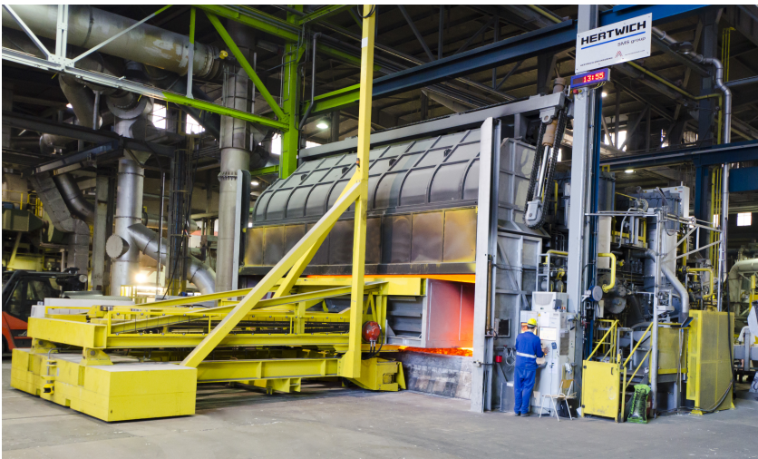
Melting and Casting Furnace (70 tons) at AMAG, Ranshofen
